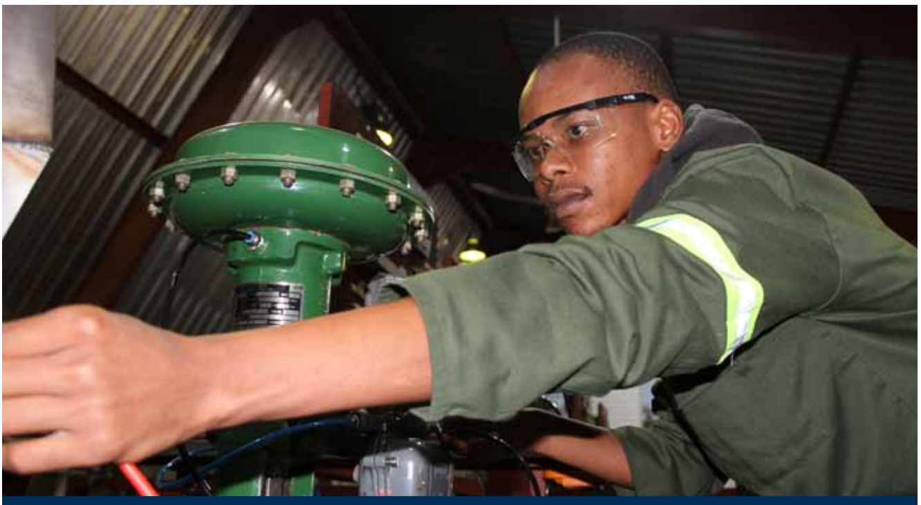
» Themba Sibeko, Control & Instrumentation Apprentice doing adjustments and calibrations on a fisher valve.
